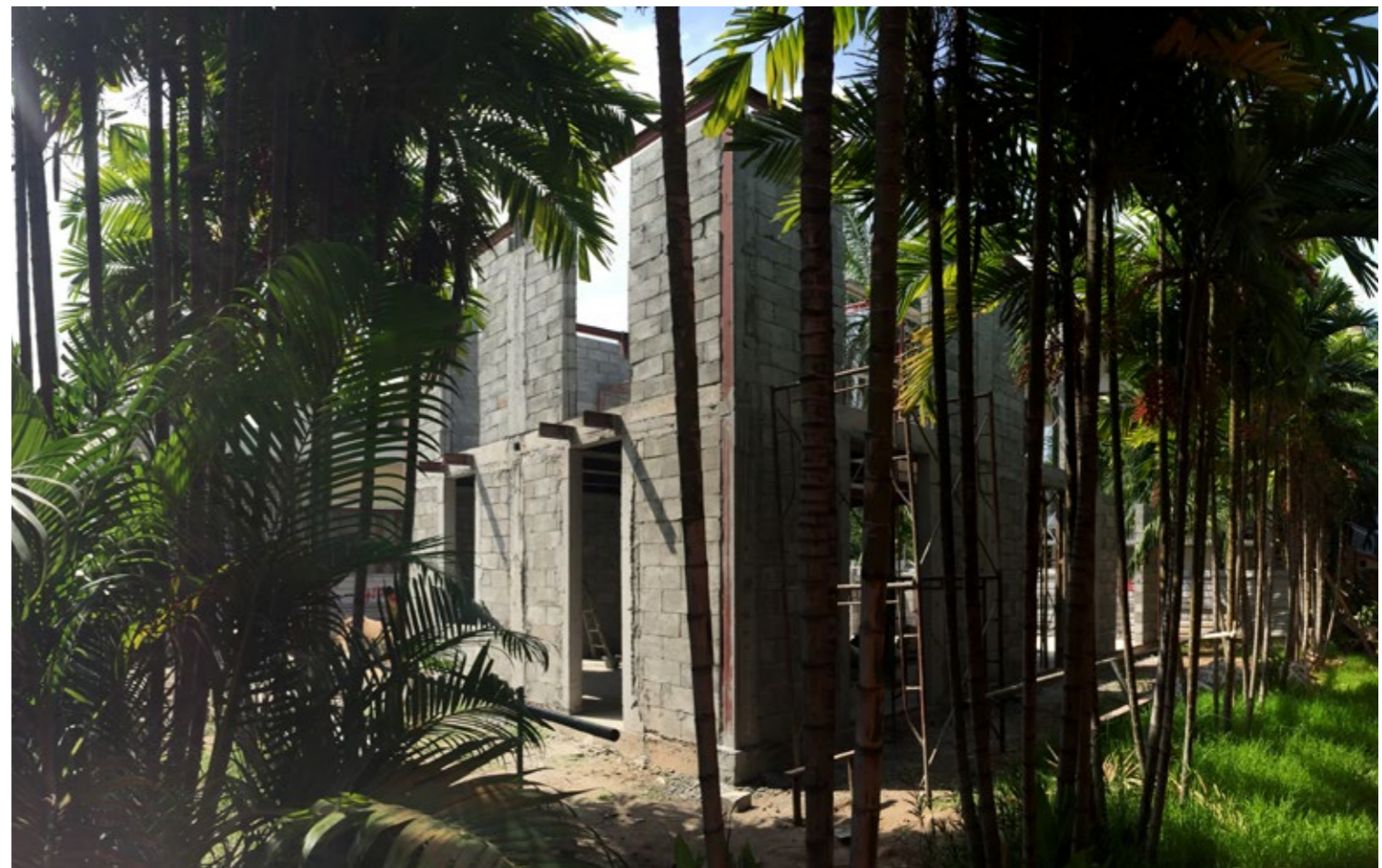
Steel structure is constructed for both floor levels including roof. Pre-cast concrete panels are used for level 2 base flooring.
