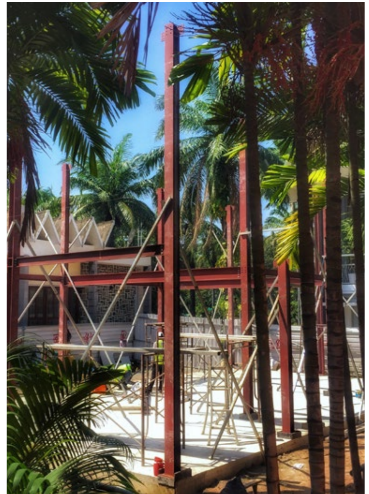
Steel structure is constructed for both floor levels including roof. Pre-cast concrete panels are used for level 2 base flooring.
